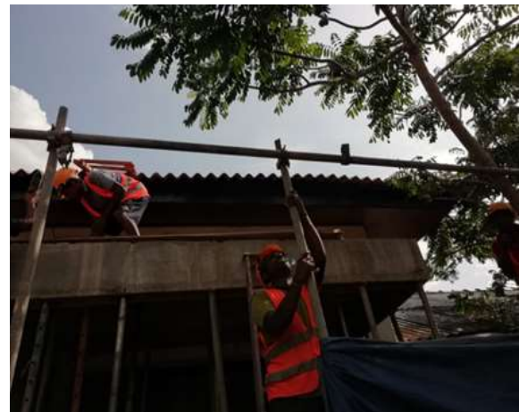
Safety for workers
