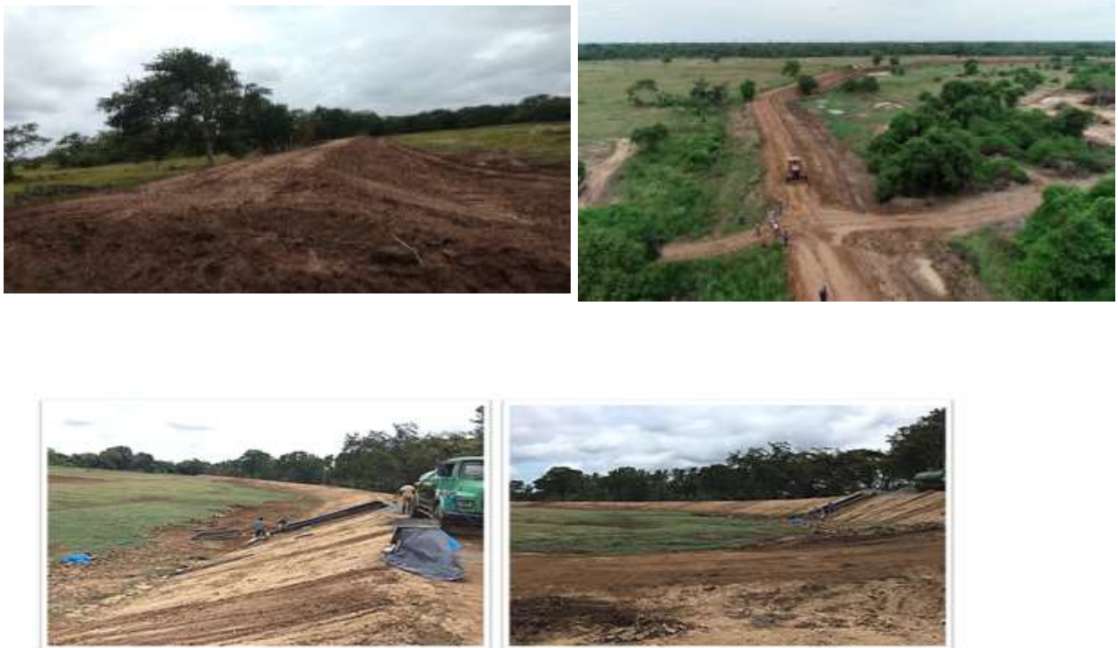
Figure 17: Ranorawa Tanks under construction
