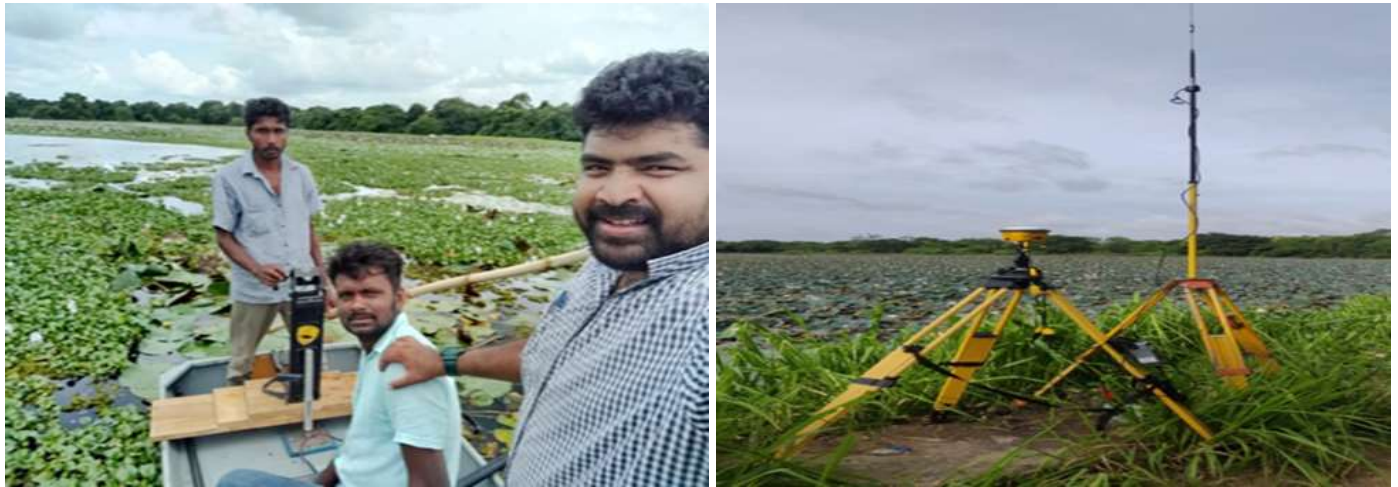
Engineering Survey is in progress – North western
