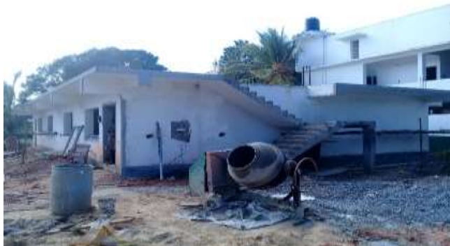
Buttala ASC -Uva under construction
